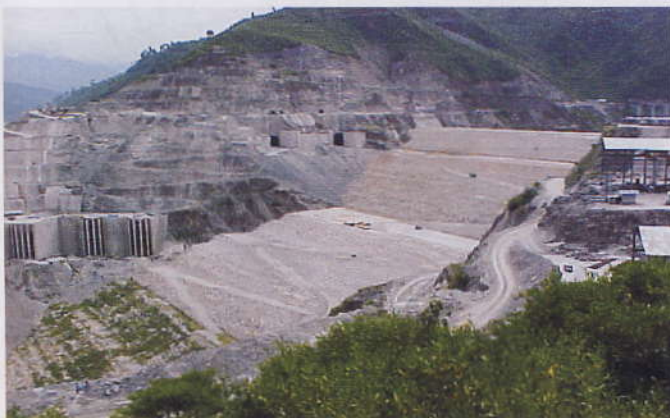
Another view of dam on completion
