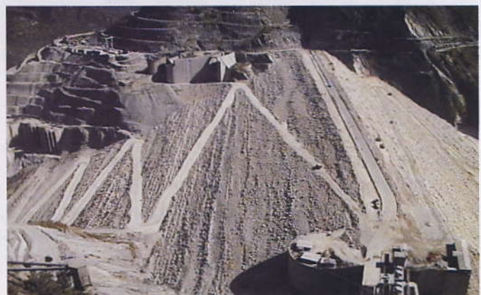
Dam after completion of construction
