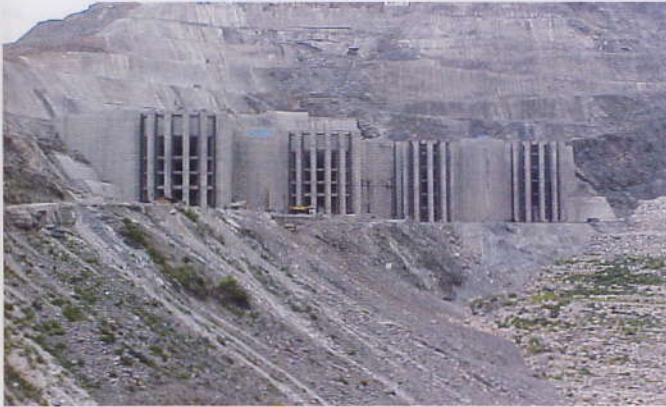
Intake structure under construction
