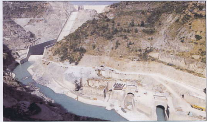
A view of the completed works from downstream side
