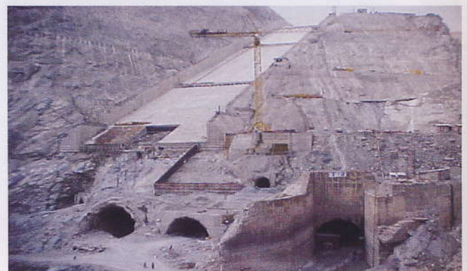
Chute Spillway under construction
