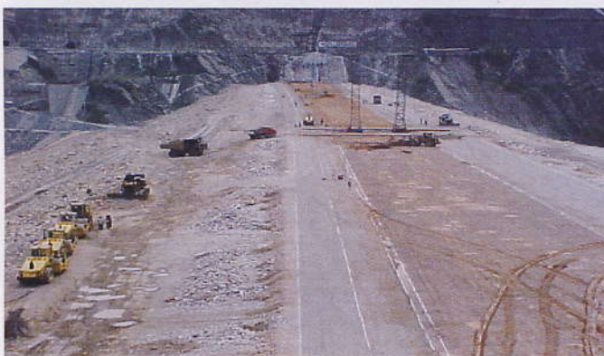
Dam under construction
