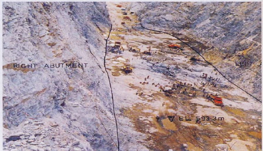
Excavation of Core Trench of Tehri Dam
